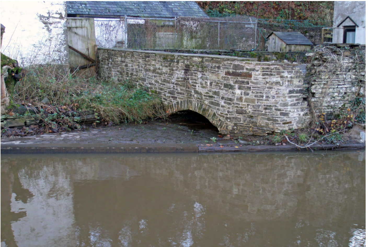
The new refurbished by-pass weir at Tyn-yr-heol Lock
