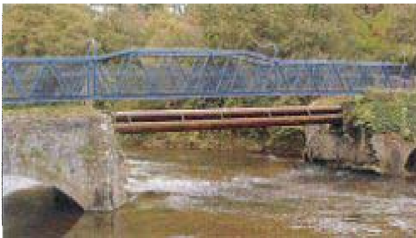
The flood damaged aqueduct at Ynysbwlllog with the temporary footbridge
