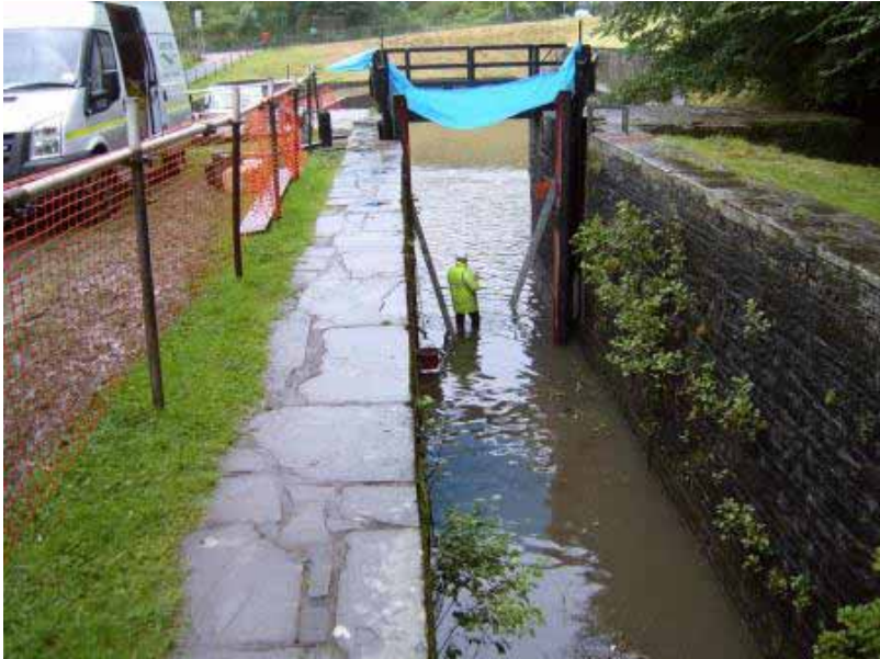
From the archives – Replacing the Lock gates at Resolven.
