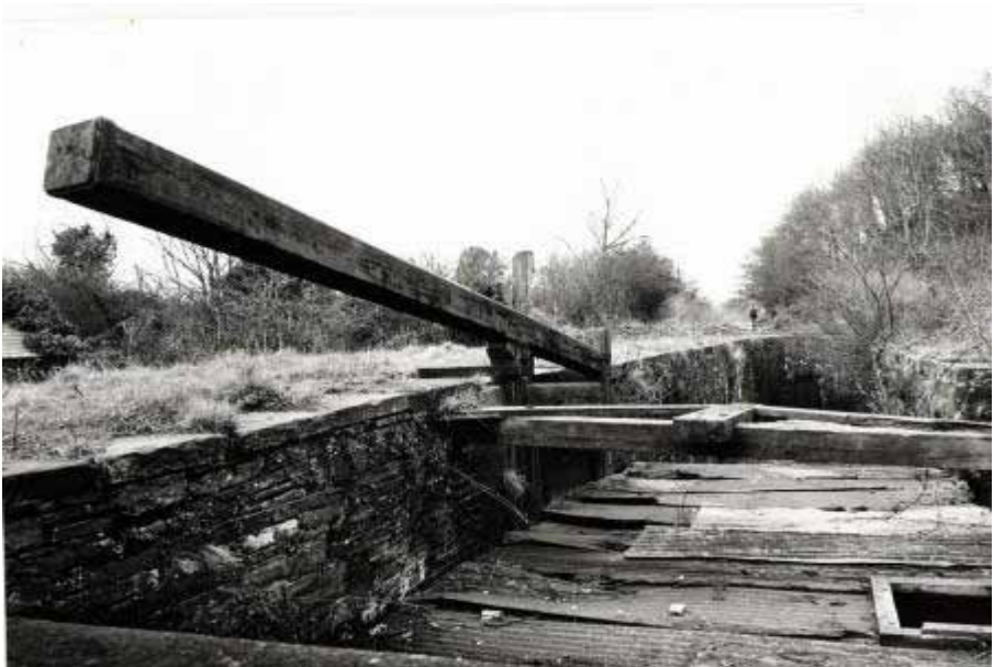
Before Resoration – Lock at Clyne (above) Lock at Tonna (below)
