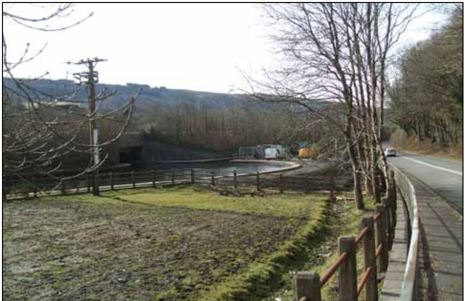
Access improvements near Ynysbwllog Aqueduct.
