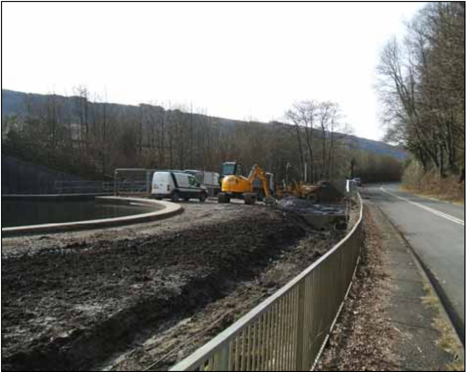
Work in progress on the Neath Canal near Ynysbwllog Aqueduct.
