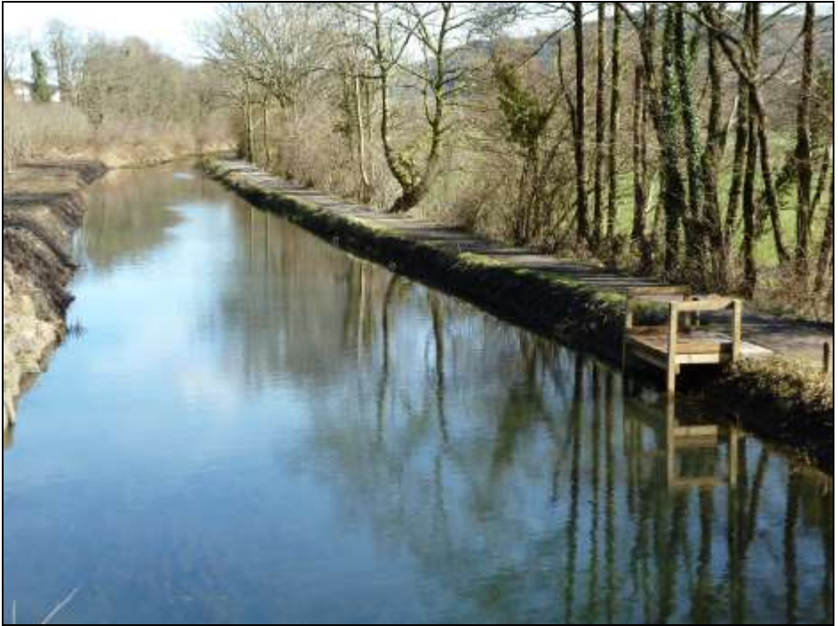
The Neath Canal at the Waterways Festival site – Ynysawedd Farm. Note the new landing stage. The festival site will be on the fields to the right of the photo.
