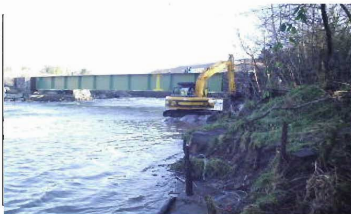
Ynysbwlllog Aqueduct – looking up-stream
