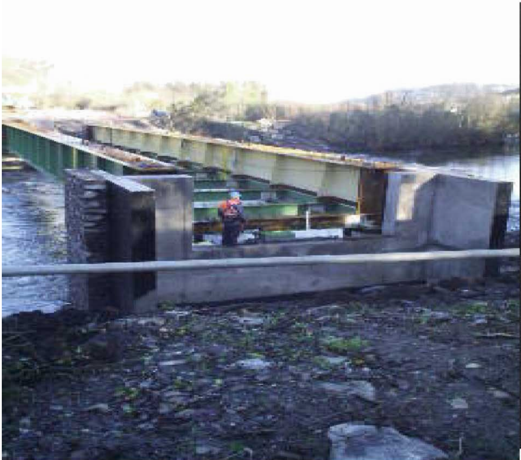
The new Aqueduct at Ynysbwllog takes shape – December 2007.
