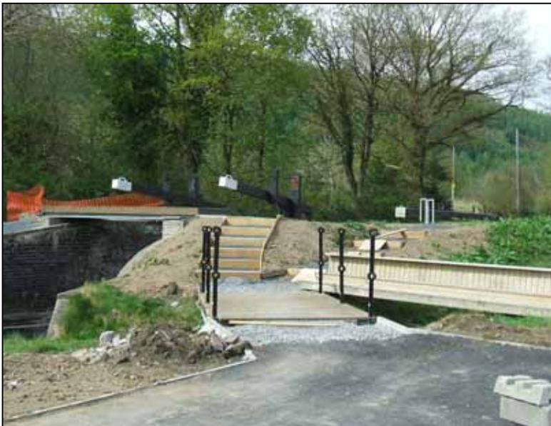
Clyne Lock – building new bridges across the lock and bypass weir.
