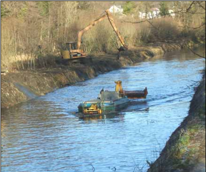
Improvement work on the Neath Canal at Ynysarwed – Dec 2010.
