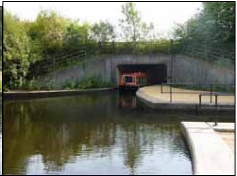
The A465 Bridge
