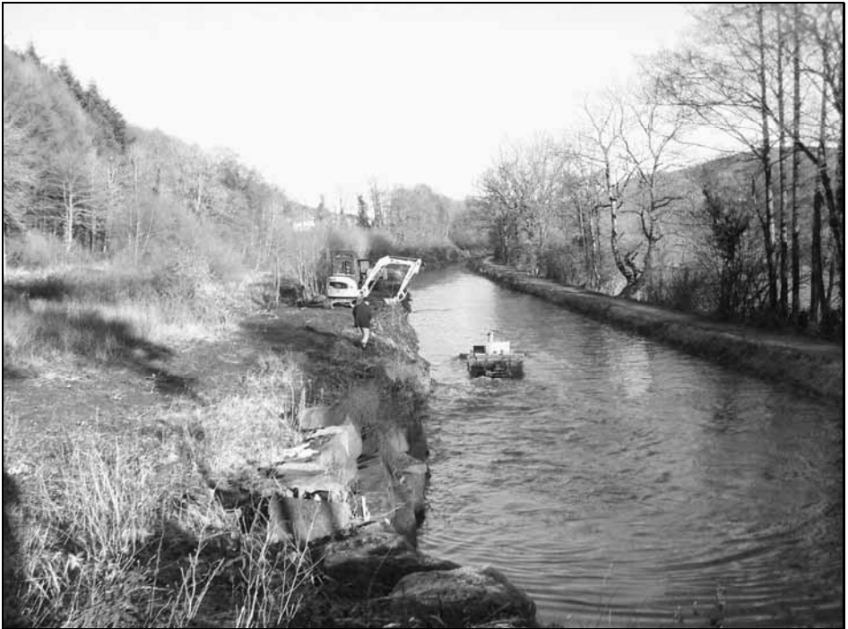
Canal improvements at the Festival Site – December 2010
