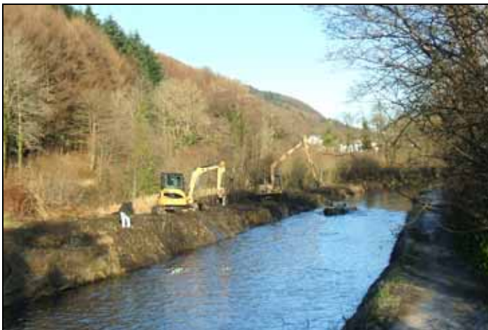
Work in progress near Ynysarwed Farm – December 2010
