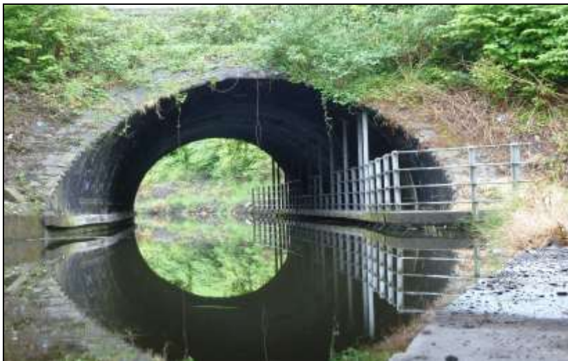
Tennant Canal - no room for a towpath so build one out over the canal!
