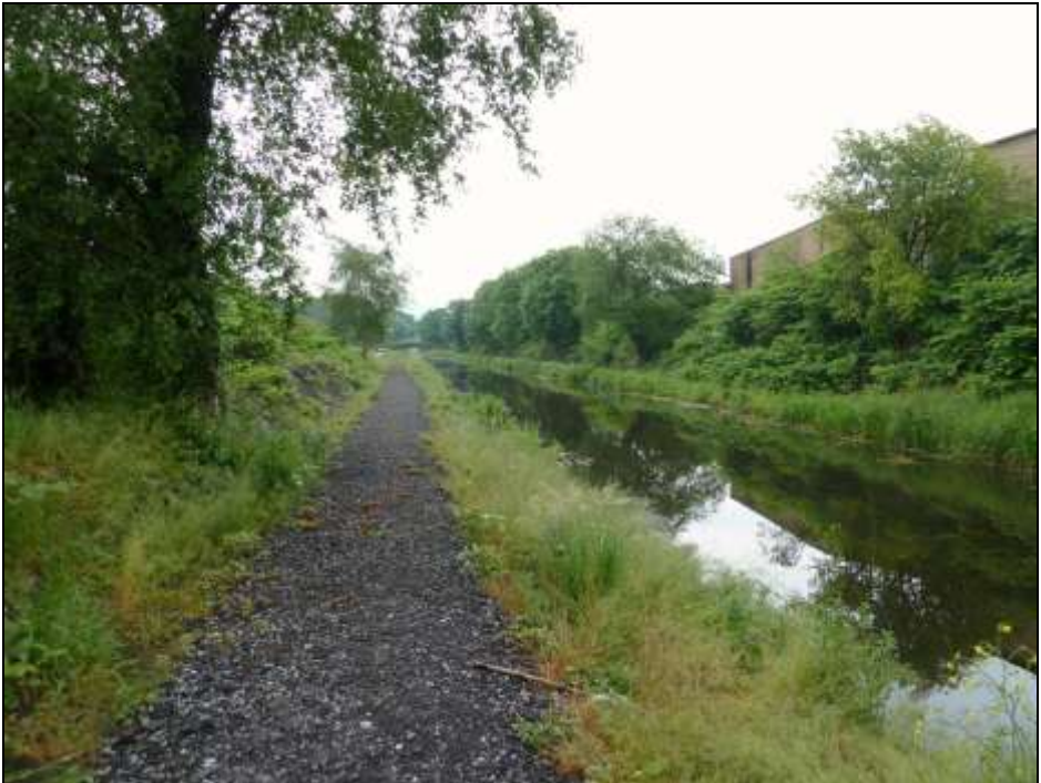
Towpath improvements on the Tennant Canal – west of Neath Abbey.
