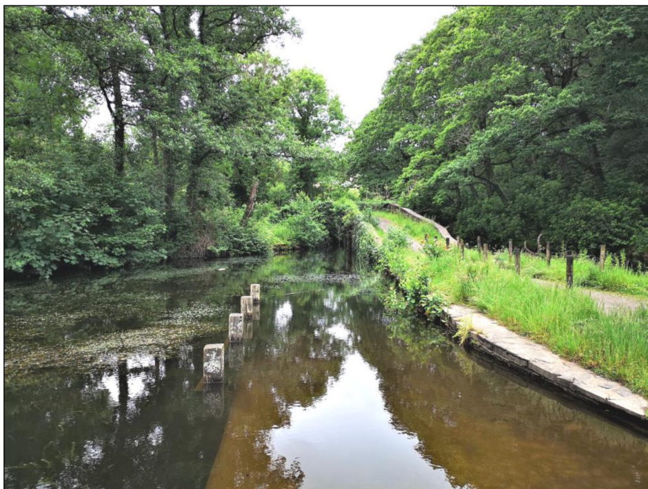
Skew Bridge. Aberdulais Basin, disappearing under ivy and saplings.
